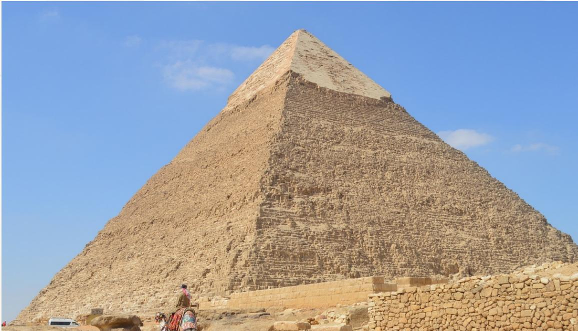
This is what is left of the limestone casing that would have covered the whole pyramid.
