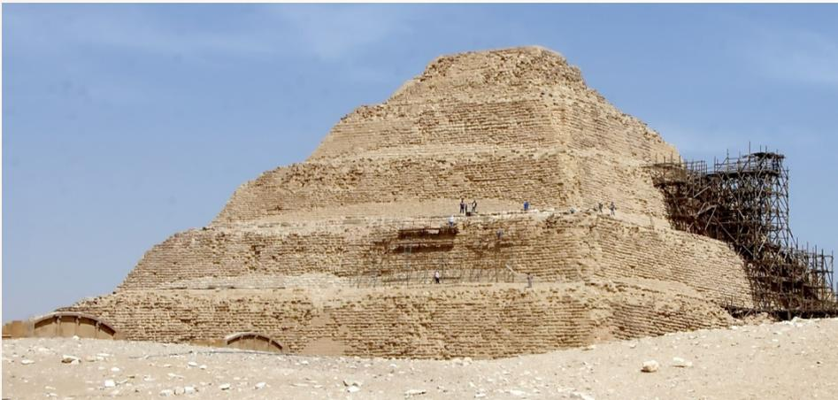
Similar to the mastaba, the burial chambers of the step pyramids were underground and complex. However, tunnels and passages of the Djoser were lined with limestone instead of wood.
