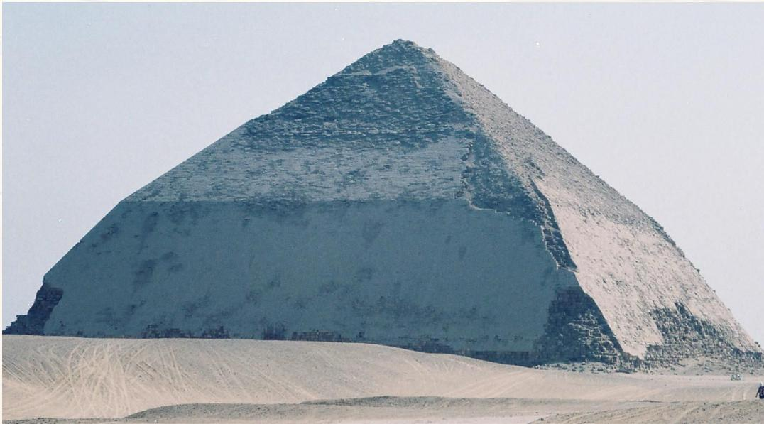
However, when the building began, the  $55^\circ$  angle of the slope was too steep and while building, engineers realised it was unstable. So, half way up, the angle was changed to  $43^\circ$  to make it more shallow.
